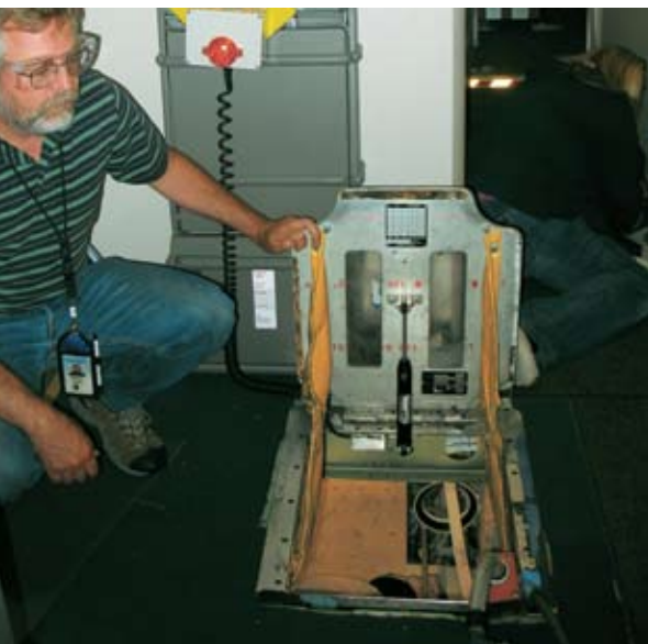
This hinged, self-closing E/E bay main deck access panel is used during 777 production. Note that the panel is connected to a red light, which flashes any time the access panel is open.
